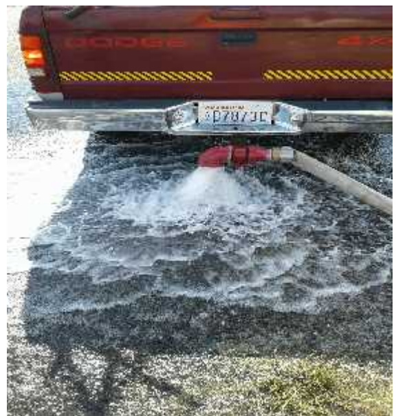
< Blow Off being flushed on Sunridge Ave.
